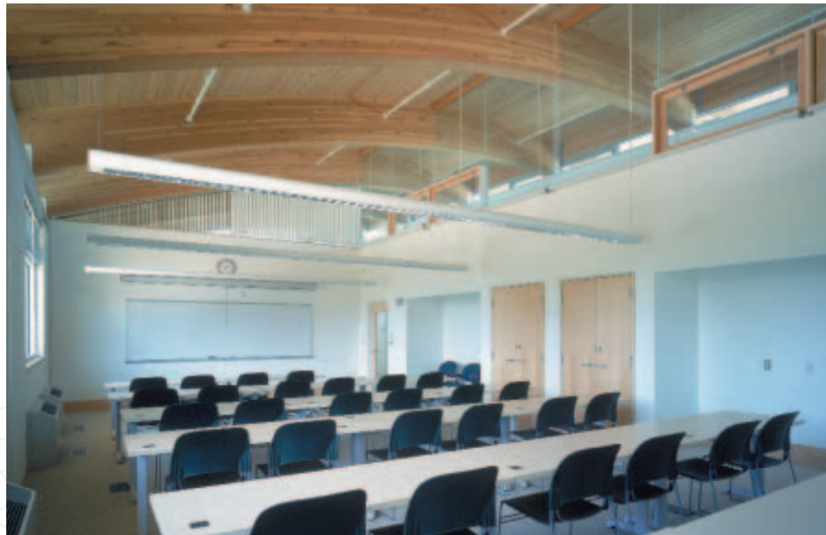
Direct/indirect lighting fixtures supplement daylighting to maintain constant luminance levels in this classroom within the Lewis Center for Environmental Studies at Oberlin College in Oberlin, Ohio.
