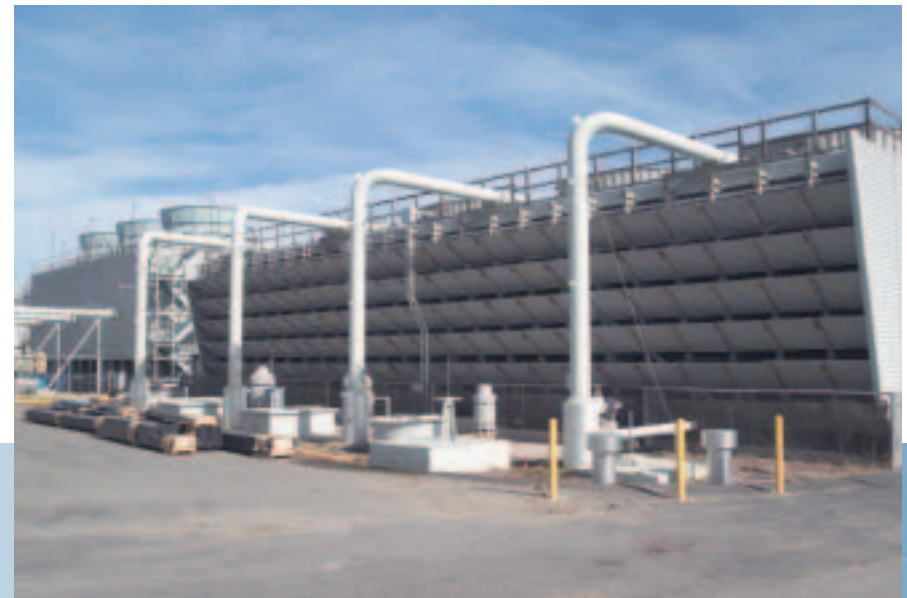
Provide variable-speed-drive (VSD) fans on all new cooling towers. A direct-drive propeller axial cooling tower is usually more efficient than a centrifugal-fan cooling tower. Over-sizing the cooling tower enables condenser water to return to the chiller at a temperature close to the wet bulb temperature, maximizing system efficiency.
