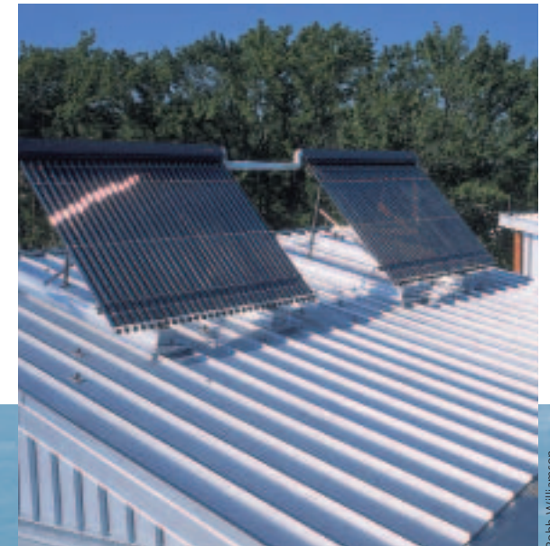
Smaller solar hot water systems, such as the system installed at the Chesapeake Bay Foundation's Philip Merrill Environmental Center in Annapolis, Maryland, are more common than larger systems, such as that found on the LANL Otowi Building.
