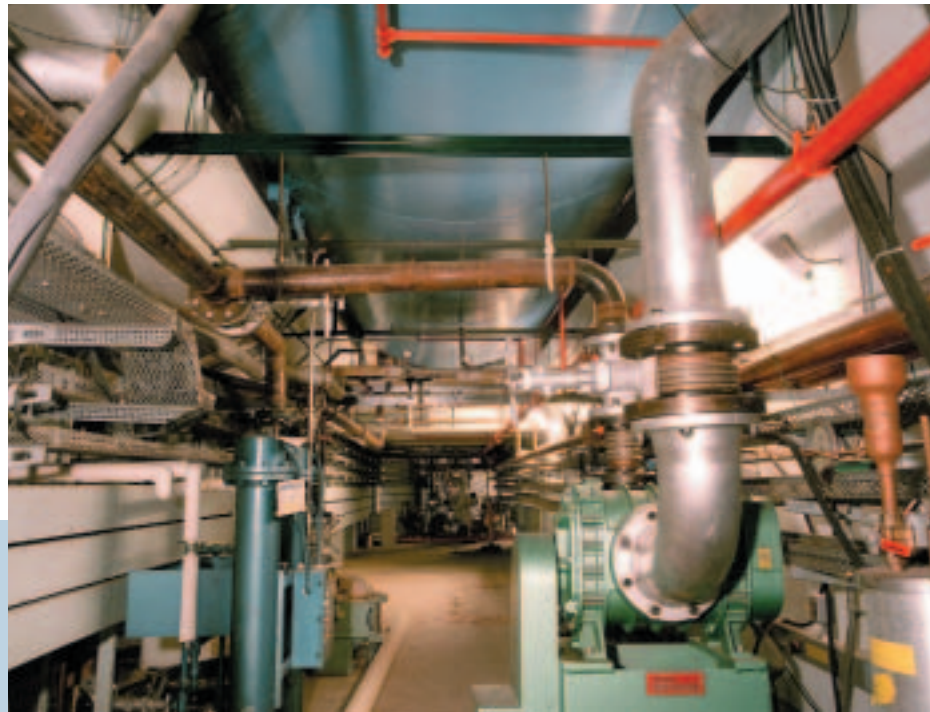
The LANL Ion Beam Facility mechanical room.
